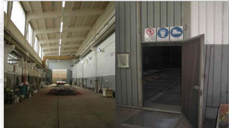
Shot blasting area
