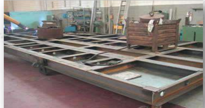
Structures construction and welding
