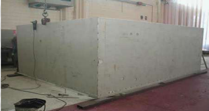
Tank construction and welding
